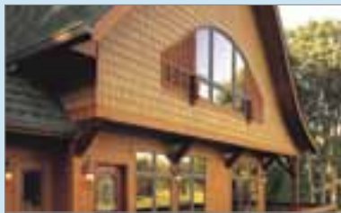
Fiber Cement Siding
